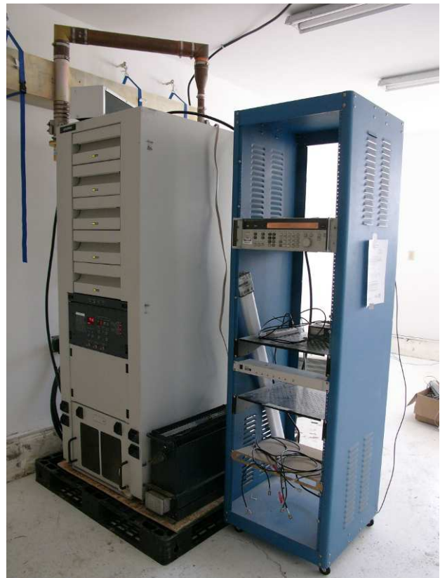
Figure 2: 2 kW transmitter donated by KUTV-2, in operation at Millard County, UT Cosmic Ray Center.
