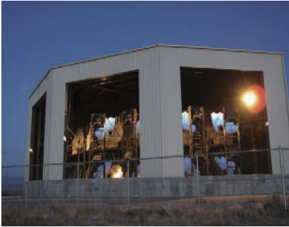
Figure 7. One of FD station (Black Rock Mesa)
