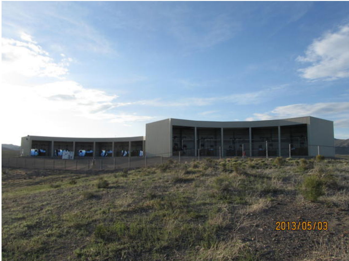
Figure 2.15: Photo of the MD (left) and TALE (right) telescope buildings with opened shelter doors. The shorter main TA building contains 14 telescopes viewing 3\text{-}31^\circ elevation. The taller building on the right has 10 TALE telescopes viewing 31\text{-}59^\circ elevation above the field of view of the main TA telescopes. Reprinted with permission from J. N. Matthews.
