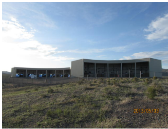
Figure 2: The lower building on the left is the main TA building contains 14 telescopes viewing 3-31° elevation. The taller building on the right has 10 TALE telescopes viewing 31-59° elevation above the main TA telescopes.
