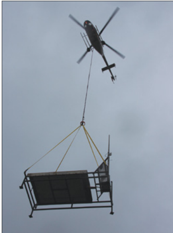
Upper Left: Cosmic ray detectors waiting to be transferred to permanent positions. Lower Left: A cosmic ray telescope works in conjunction with the detectors. Right: The detectors are air-lifted into place with helicopters.
